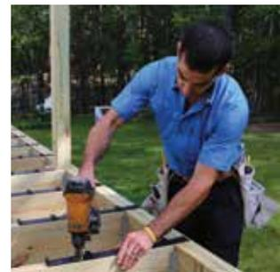
The strip protects the top of the joist from water damage, rot, and decay.
